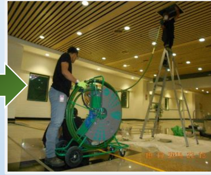
AIR DUCT CLEANING
