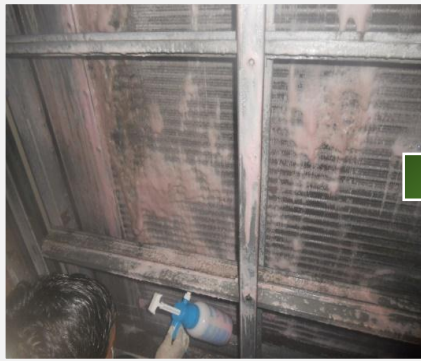
AHU CLEANING & TREATMENT (COIL TREATMENT)
