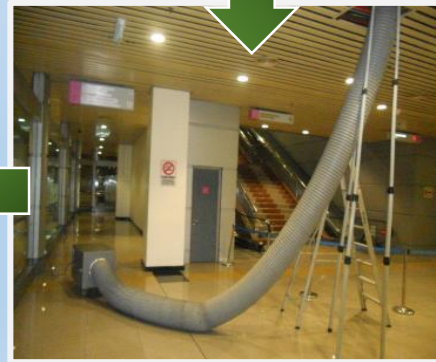
PROCESS TO REMOVE DUST & DIRT FROM INTERNAL DUCTING
